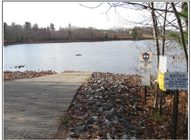
The State boat launch was pretty much unusable last fall except for carry-in traffic. There is less than 2' of water by those rocks.
