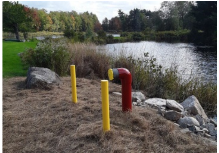
There is now a dry hydrant over at the Clary Lake dam. Many thanks to David Boynton for donating his time!
